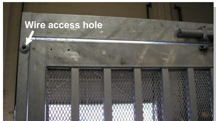
Figure 3 The wire access hole as indicated by the arrow. Left hand orientation from push bar shown.
