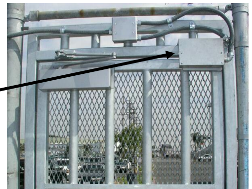
Figure 4 Magnetic Lock box shown from left hand orientation from push bar.
